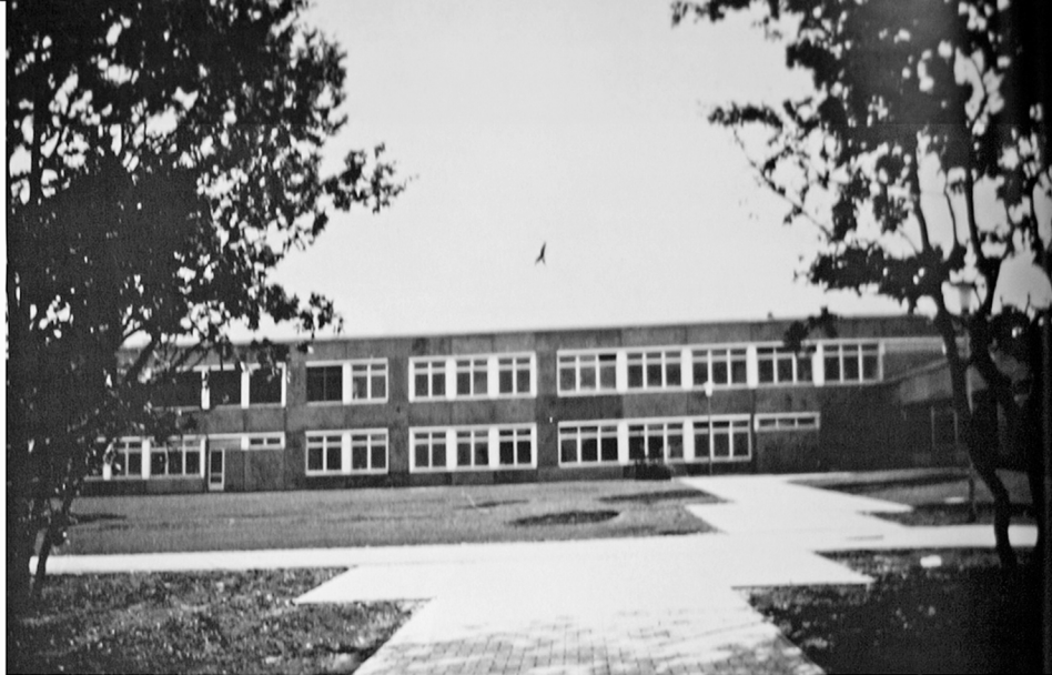
Bitburg Gets New High School for 1975-6, Cooperation Brings Building in Record Time
